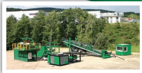
Site set up.
